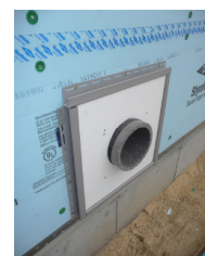
Mounting block installed over Roflex gasket
