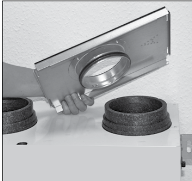
2. Attach end plate to CA 200
