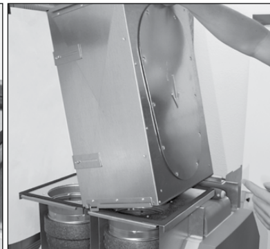
9. Place ComfoWell on the end plate
