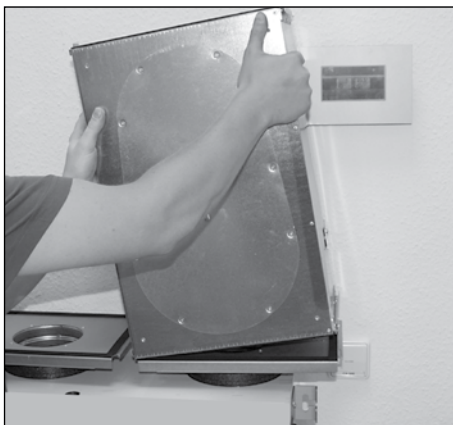
4. Place attenuator on the end plate
