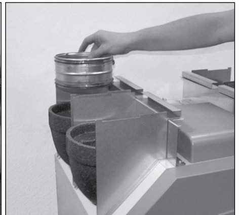
6. Insert the 160 mm nipple into the CA 350
